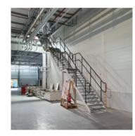
Built and installed stairs: following the blueprint drawing with a tilt of 43.39°
